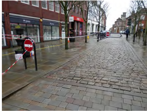
Plate 8.8 Low kerb line and reinstated setts in Market Place
